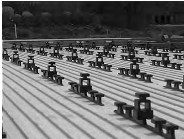
Pour concrete and allow to cure before tilting the wall section. The result is four inches of concrete on the inside and 2.5" EPS insulation on the outside. The furring strips are already in place. The wall is immediately ready to finish as required. The result: a finished wall with R-11 insulation.
