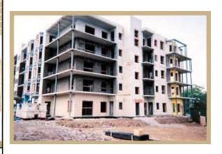
"Because of the packaged block, they were able to hoist an entire floor of block on to the floor area. With other ICFs that come made, you could not fit the entire floor on the lift, which increases hoisting costs. We were able to go from an 8" wall to a 6" wall at a corner, thereby eliminating a 2 1/2" step return. This is aesthetically pleasing and can also save the owner a lot of concrete."
