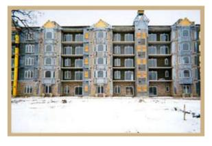
ECO-BLOCK buildings consistently save 25 - 50% in monthly utility costs over the life span of the structure, translating into fewer resources consumed for the creation of energy. Beyond the insulating qualitites of the foam block (R-22), the thermal mass of concrete acts as an energy reservoir. This helps maintain an even indoor temperature. Consequently, the HVAC system can be scaled down up to 35%, offering another added cost savings.
