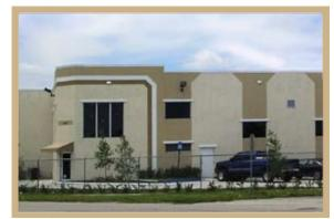
Marathon Mold's 24 foot walls were constructed using ECD-BLDCK along with steel framing & masonry. A Durolast white membrane room was added to the 8,600 square foot building. Composed of 5 inch light weight concrete, 1 inch insulation board, and the membrane, the roof sits on top of steel trusses with a metal pan deck. A stucco finish was applied to complete the exterior to the desired look.
