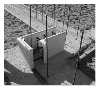
Cut the forms that butt up to a door buck, meet under a window or in the middle of a wall as necessary.
